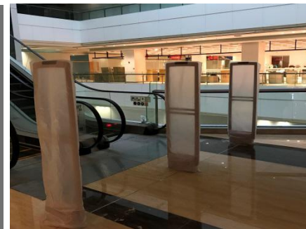
Project: Anti-theft Channel Port Installation: 2017
