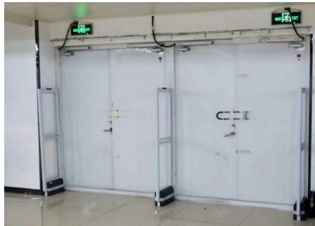
Project: Anti-theft Channel Port Installation: 2018
