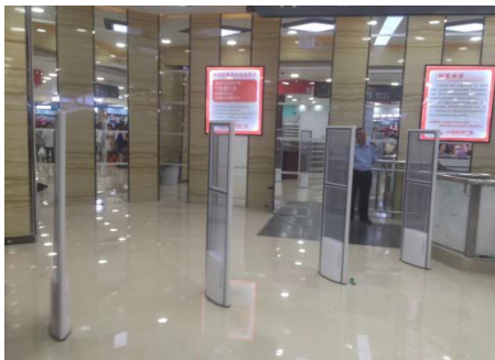
Project: Anti-theft Channel Port Installation: 2017
