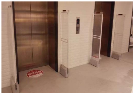
Project: Anti-theft Channel Port Installation: 2017
